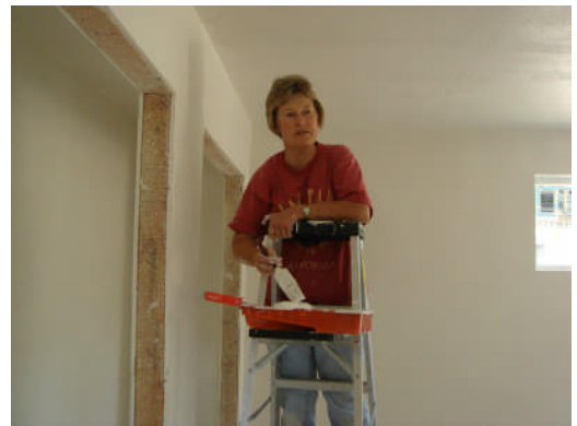
Climbing high at the Habitat house.
