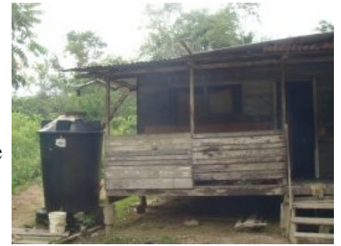
Photo of rainwater Collection device In Rwanda
