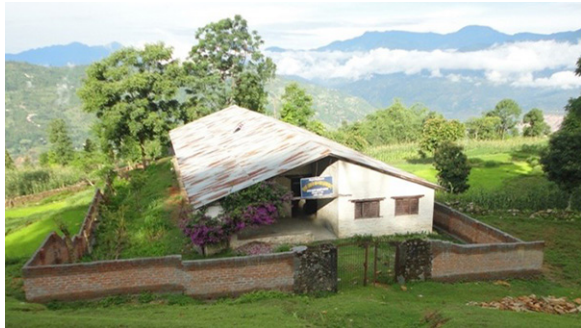
The dormitory with its new security wall.
